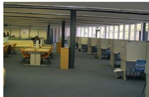
CamassCrete installed in educational institute and library. Accommodate all international brands' floor boxes
