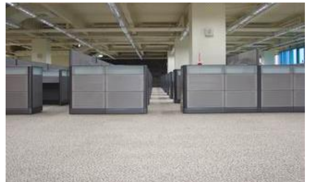
CamassCrete facilitates neat, efficient environment. Unlimited cable highway networked underneath
